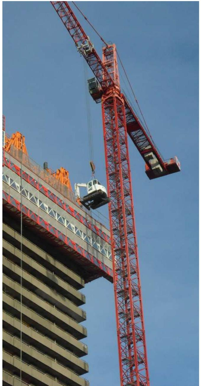
Restrictions should be placed on jib lengths to prevent loads being moved over public highways or adjacent properties. Alternatively, the use of slew limiters should be employed to protect adjacent property and the public. Effective communication between crane driver and the slinger/signaller is imperative and it is recommended that a dedicated crane co-ordinator is employed. Handset radio communication is recommended in preference of hand signals.
