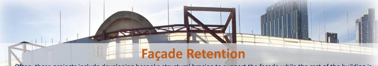
Often, these projects include developing bespoke structural bracing to support the façade while the rest of the building is being removed. Additionally, unique demolition strategies are often developed to ensure that the deconstruction does not jeopardize the structural integrity of the façade to be retained
