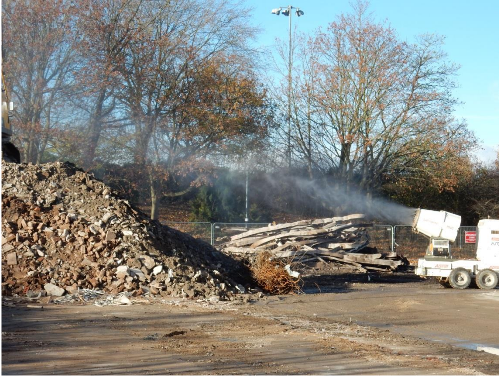
Photograph 5. Bespoke water suppression equipment.
