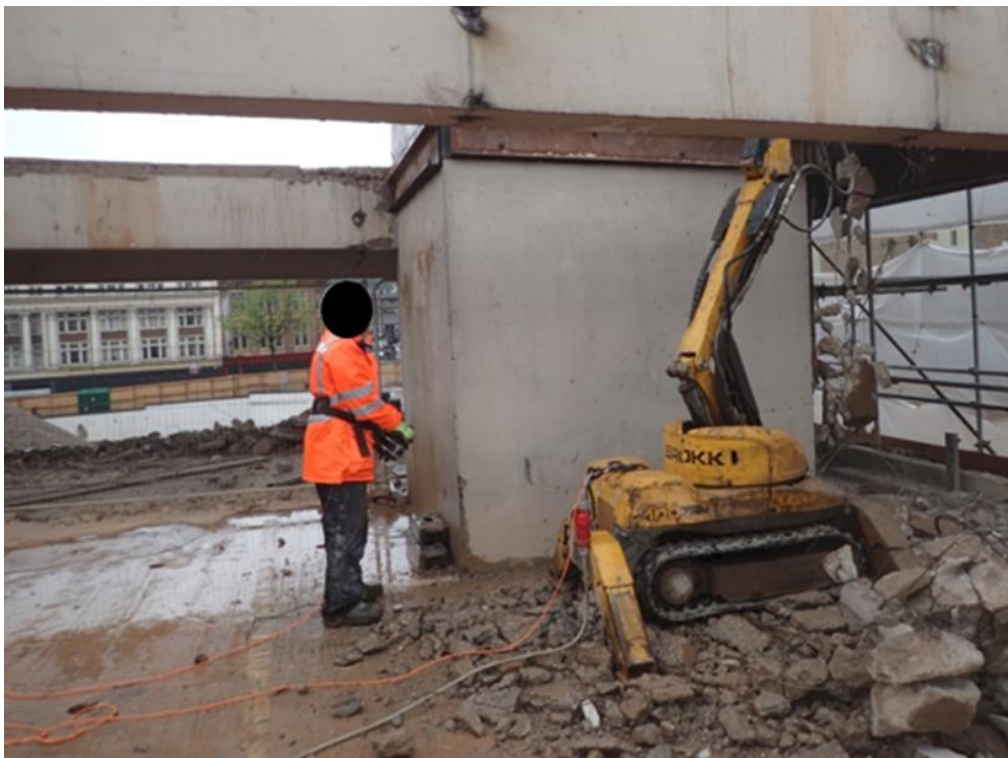
Photograph 1. Use of remote breaking equipment.
