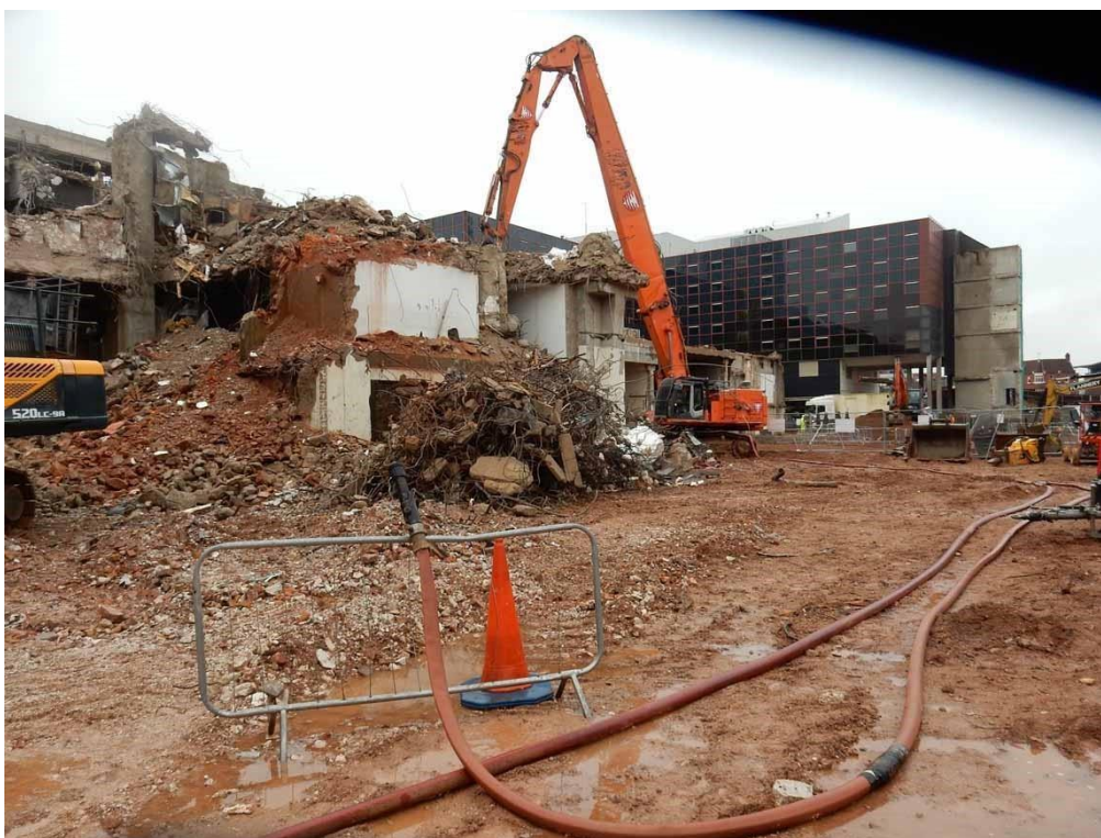
Photograph 6. High reach demolition machine.
