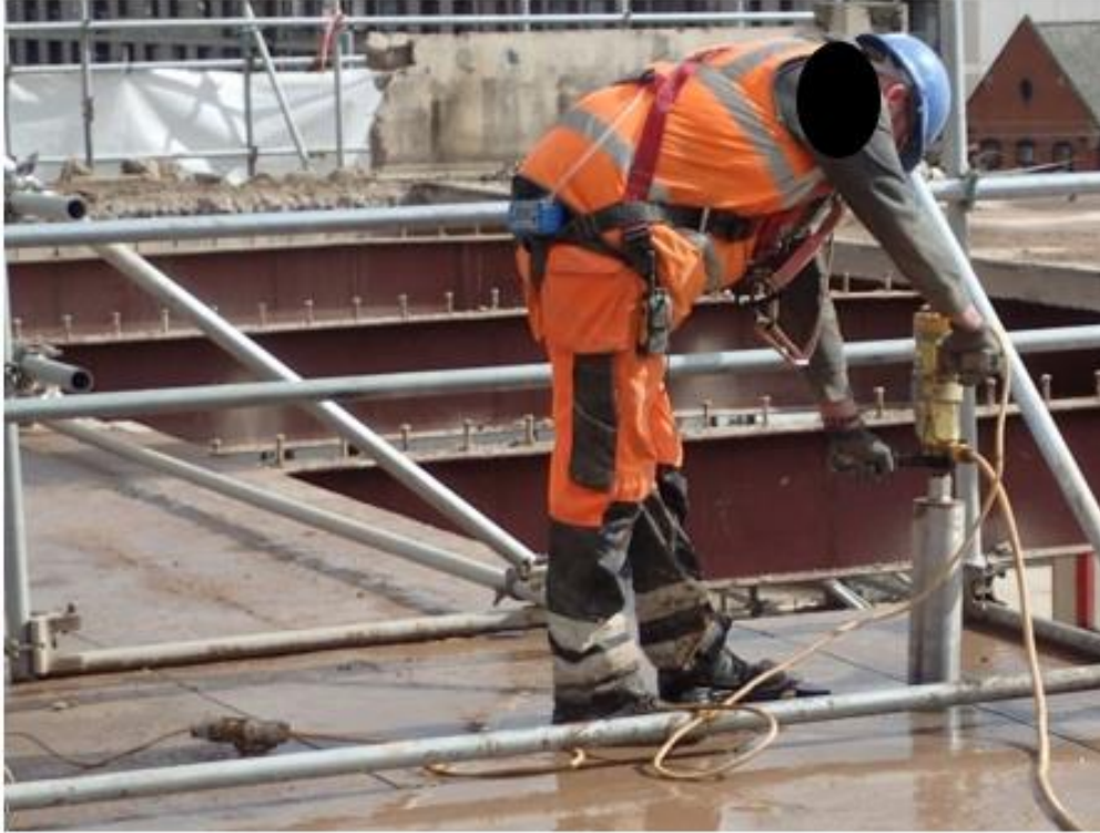
Photograph 3. Use of handheld core drill.
