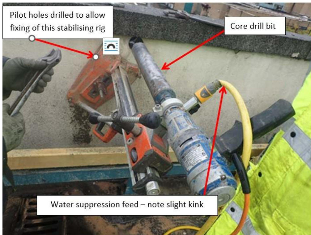
Photograph 2. Horizontal core drilling rig (bolted to vertical surface).
