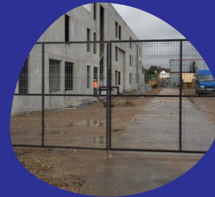
SITE ACCESS GATES
